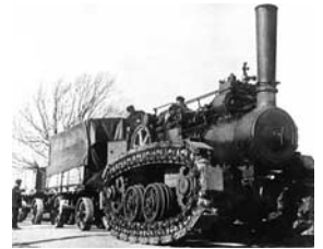
写真-15 Full Track-Laying
