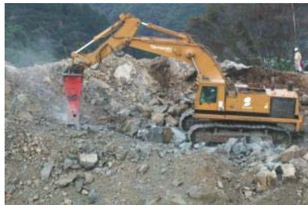
Backhoe with 5,800kg Rock Breaker (G120)
